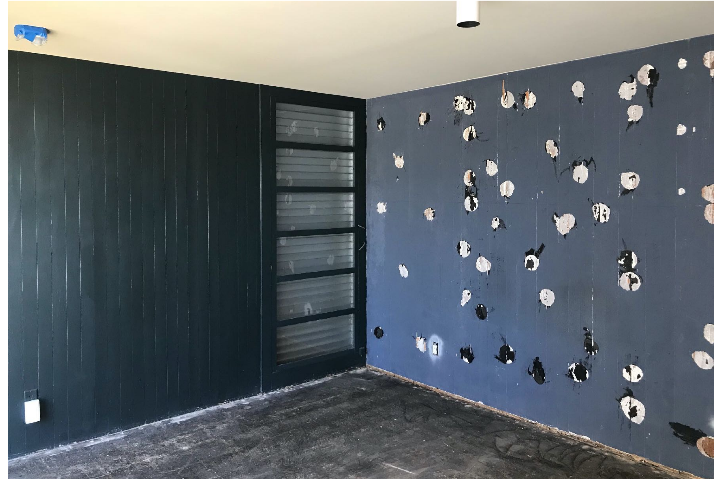
Removal of mirrored wall exposing original tongue and groove planks
