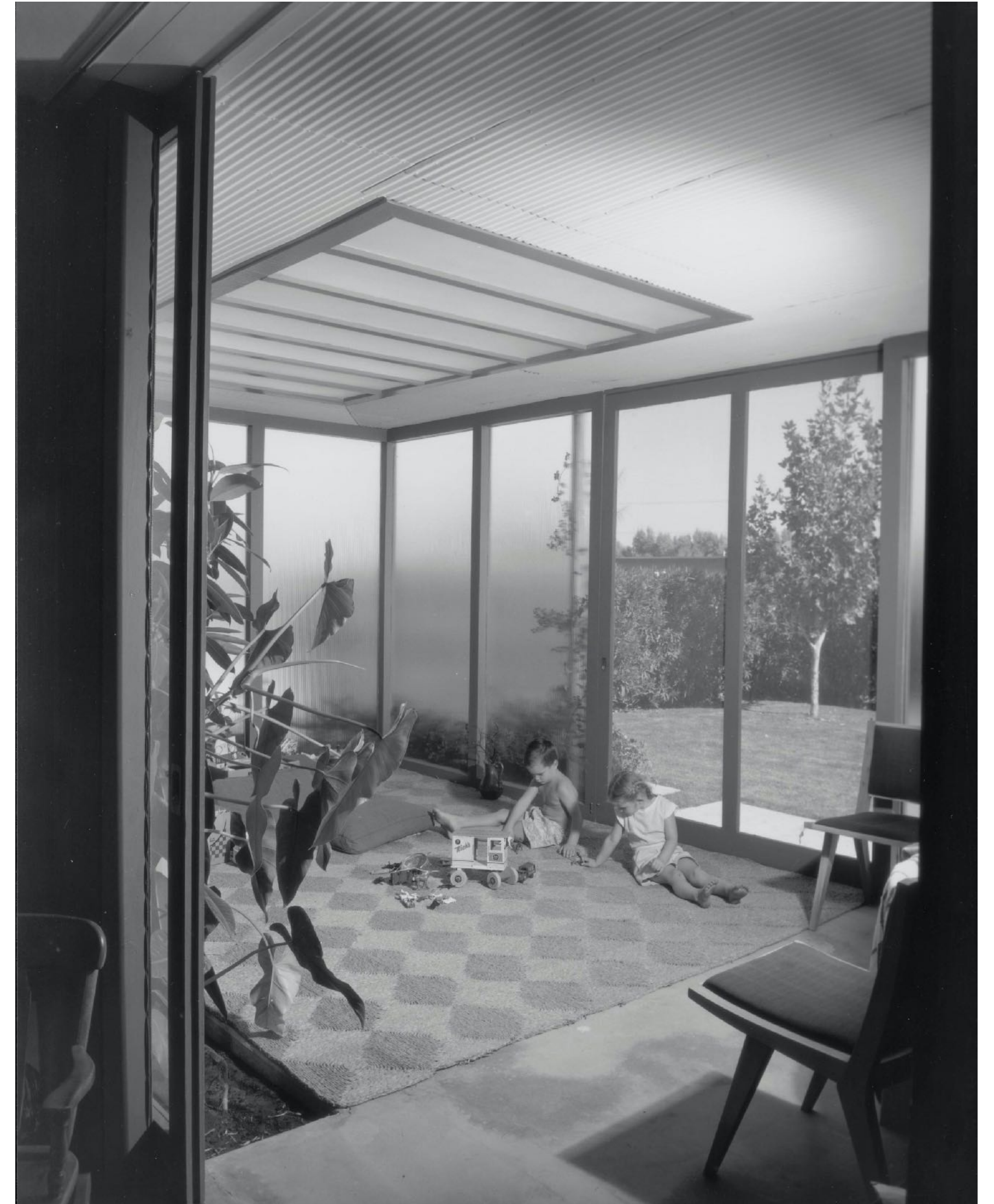
Interior of the then newly enclosed patio circa 1954
