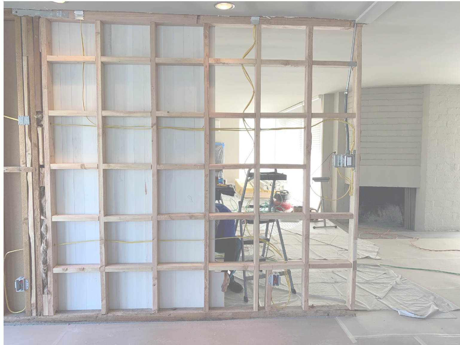
Rebuilding of structurally compromised interior fin wall
