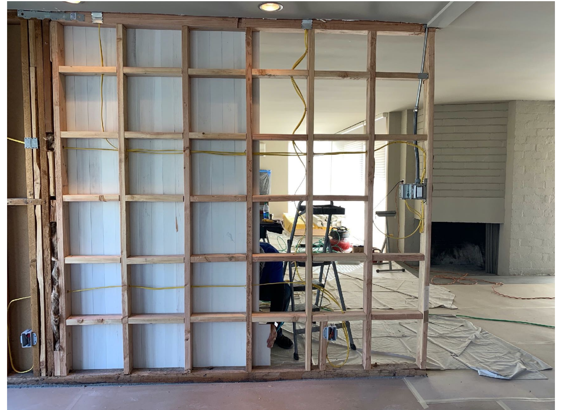
Rebuilding of structurally compromised interior fin wall
