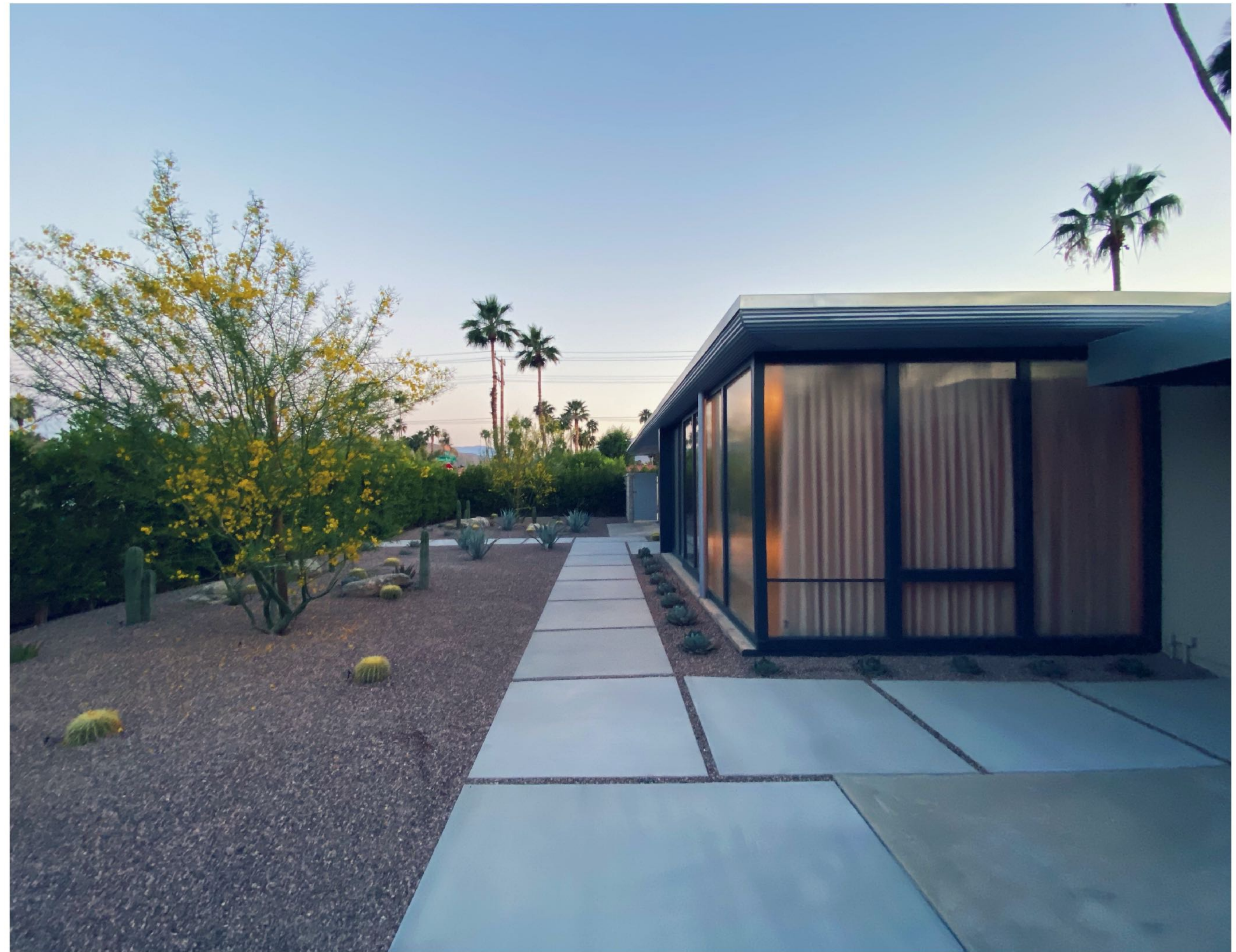
2020 view of front yard new hardscape facing south
