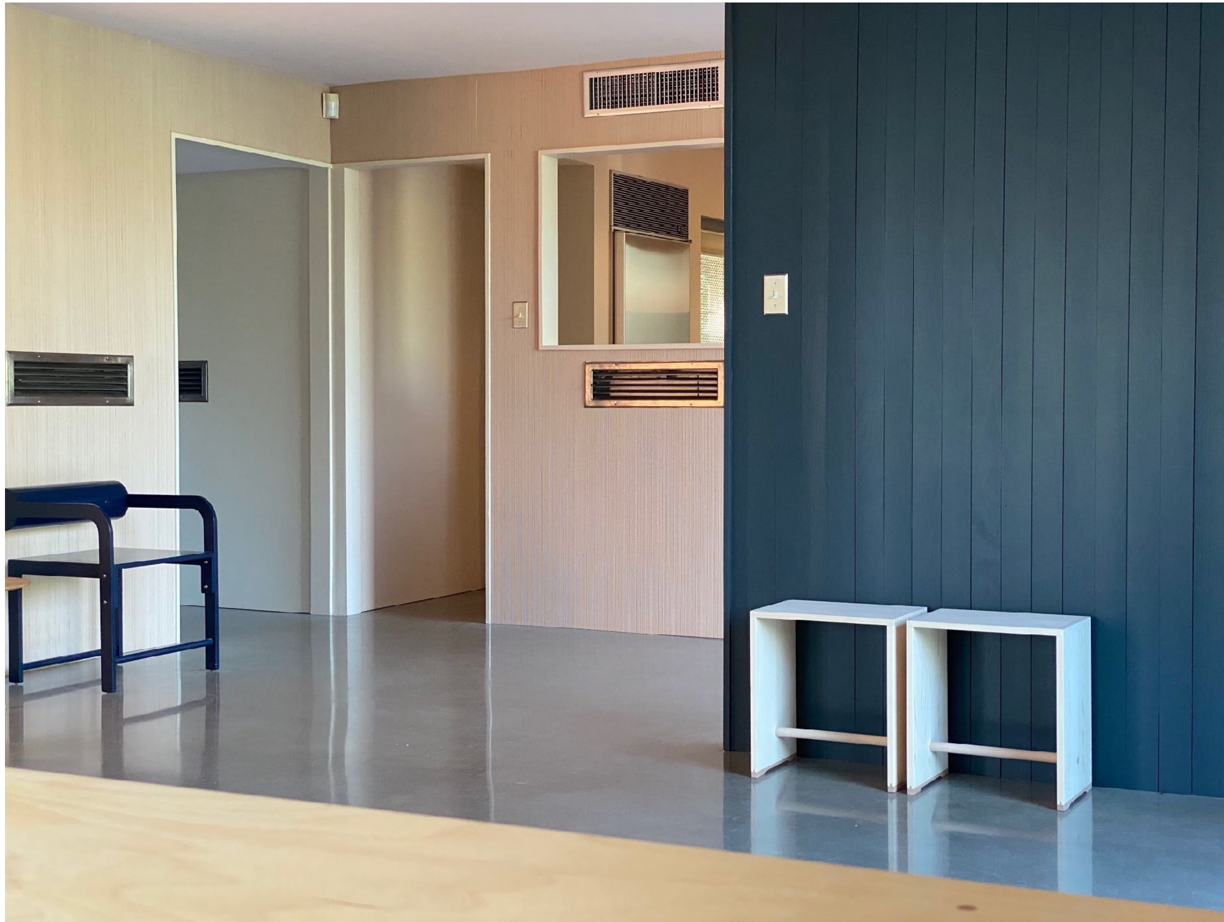
New concrete floor 2021 photo
