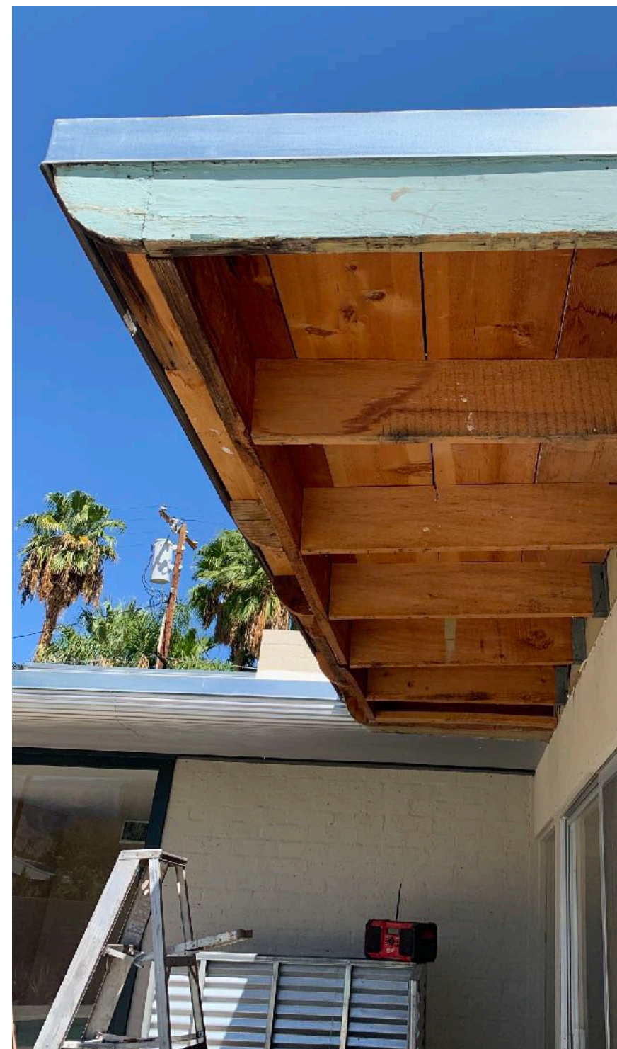
2019 replacement of sections of eaves
