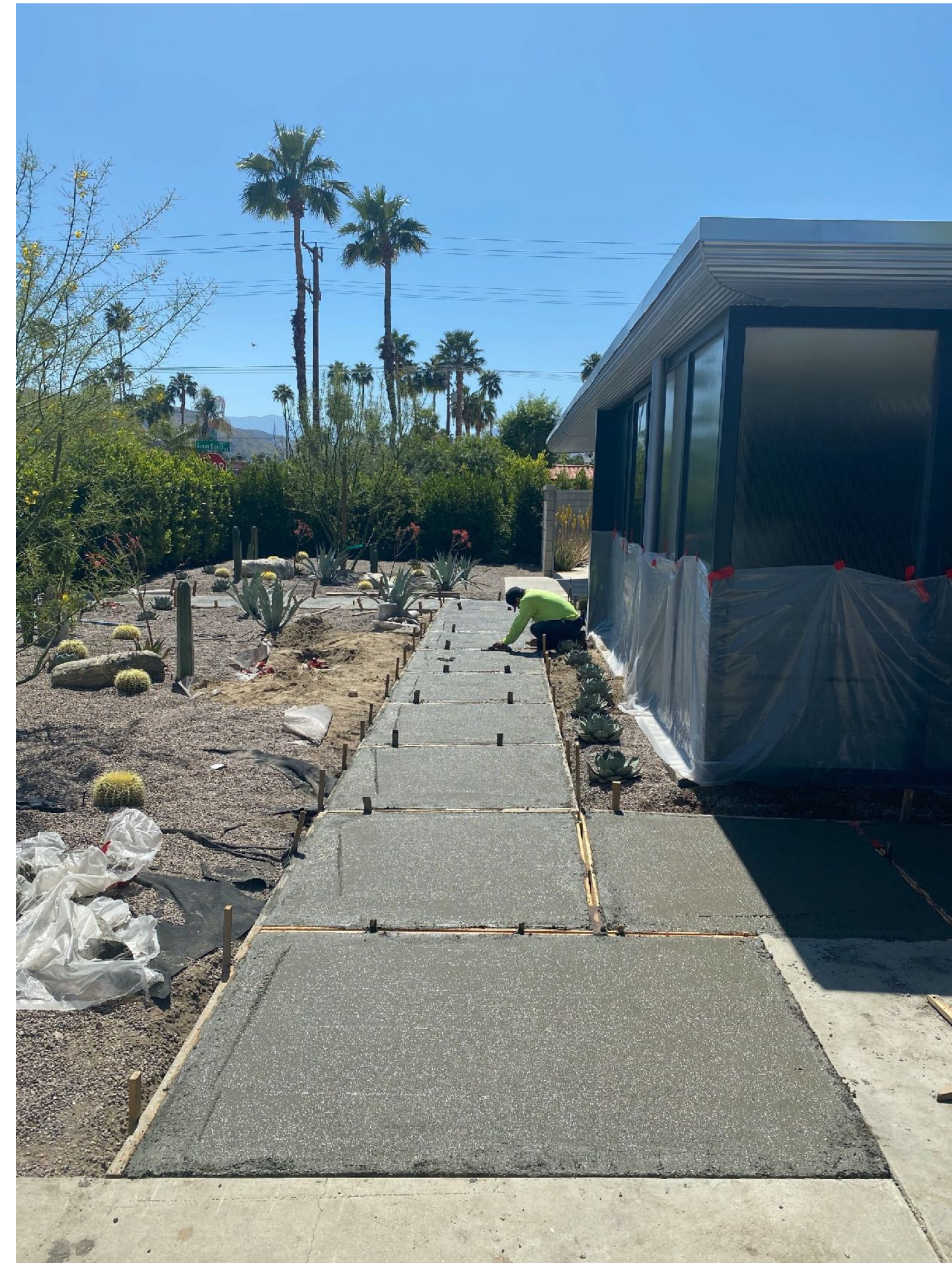
2020 restoration work in progress
