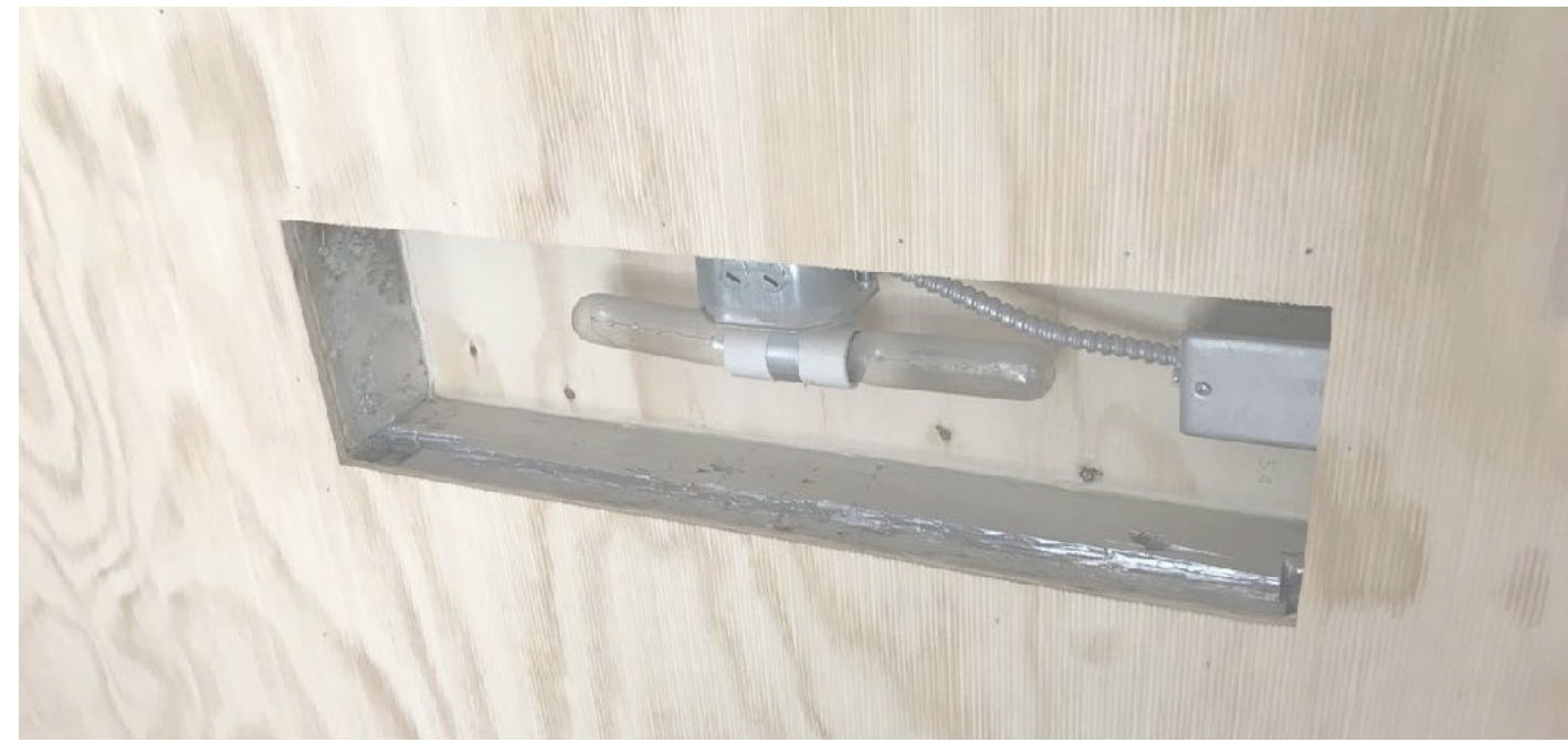
Louver light fixture exposed with installation of combed ply
