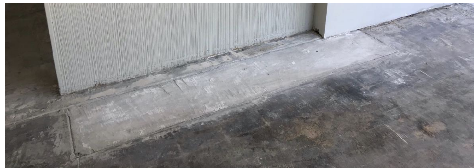
Right: tile removed and prepped For resurfacing
