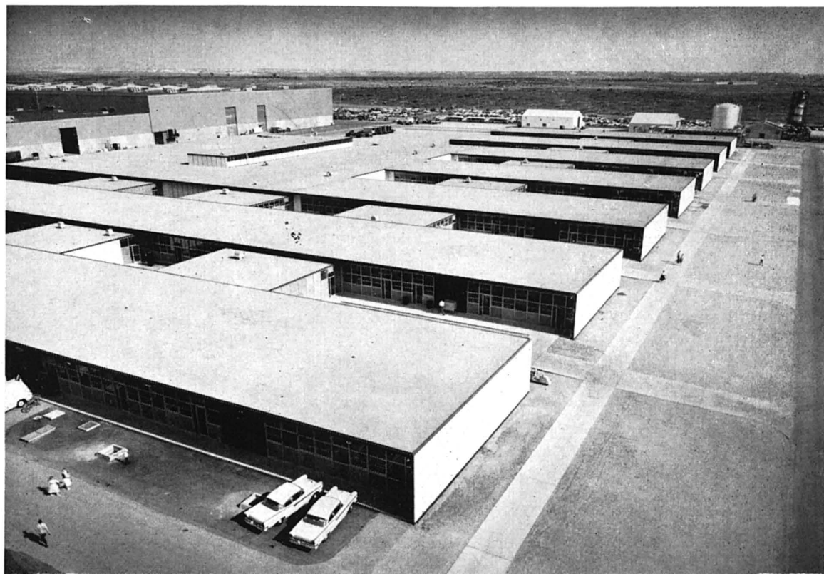
THE ENGINEERING LABORATORY IS LAID OUT IN A "WAFFLE" PATTERN. OUTSIDE WALKS ARE USED FOR INTERNAL HALLWAYS.
