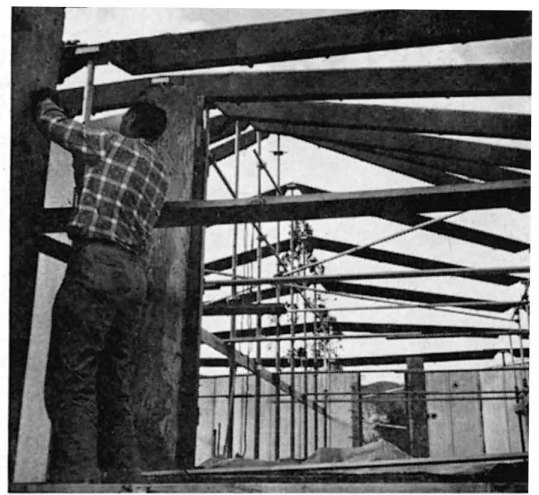
Prototype thinshell concrete roof – formed and
