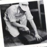
BATS which fit snugly between studdings and joists. Easily cut to fit around doors and windows.
