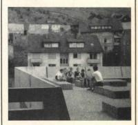
Much of the structure of the building is poured-in-place retaining walls, columns, beams, and ceiling slabs. The deep exterior parapets and fascias, however, are of precast concrete; and interior partitions are of face brick. The pleasant contrast between the roughly formed, poured-in-place surfaces and the smoothly precast parapets is one of many subtleties in detailing.
