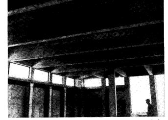
(7) Cast-in-place beams over the recreation area of the building are post-tensioned.
