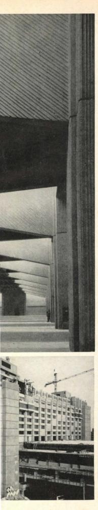
Place Bonaventure, the latest in Montreal's collection of mammoth-scaled, multipurpose urban compositions (see Sept. '66 issue), is being rushed to completion in time for this month's opening of Expo 67. The reinforced concrete structure, ribbed and sandblasted on the exterior, covers six acres of air rights over the Canadian National railway tracks and ties in with the city's underground network of pedestrian-shopping-subway facilities (section lower left.)
