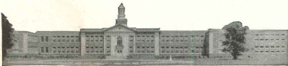
Grade School, Canandaigua, New York Duane Lyman & Associates, architects and engineers, Buffalo; H. J. Bareham & Sons, heating contractors, Rochester
