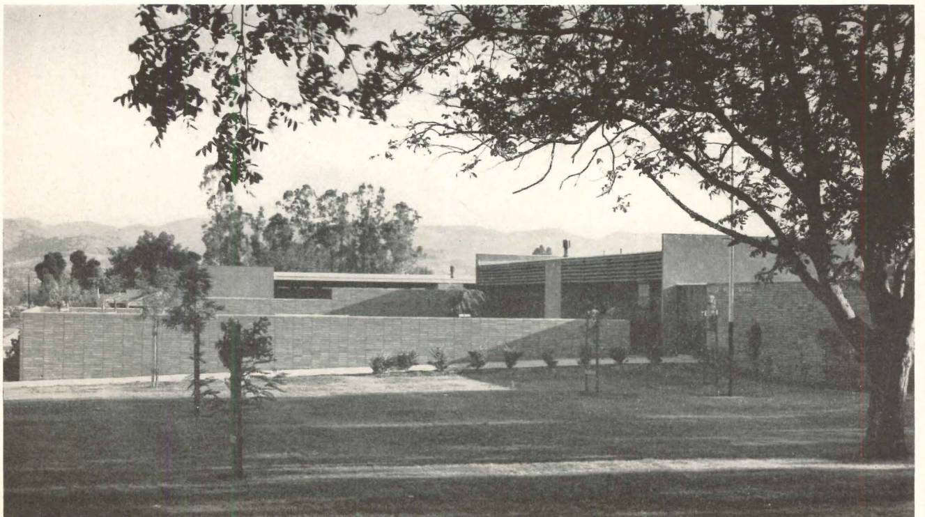
The buildings are constructed with concrete floors covered with asphalt tile. Walls are wood stud, finished with plaster or plywood. Roofs are light gravelled composition over wood rafters, ceilings are surfaced with acoustical tile. Canopies over walks (above) are supported by steel columns painted bright coral
