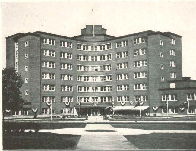
Kitchener-Waterloo Hospital, Kitchener, Ont.; Gowan, Ferguson, Lindsay, Kaminker, Maw, Langley, Keenleyside of Toronto, architects
