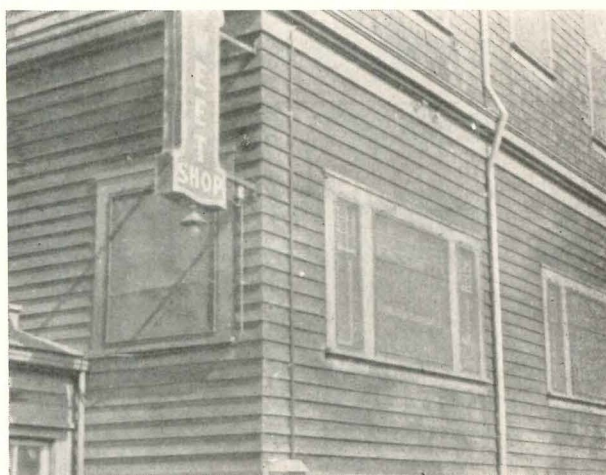
Above: Redwood Inn at Scotia, Calif., with redwood siding and trim on first floor, redwood shingles on the second. It was 20 years old here and had never been painted. Below: the Old Fairbanks House, Dedham, Mass., built in 1636 and never painted. White pine siding was replaced in 1903. Window frame, fascia wood may be the original
