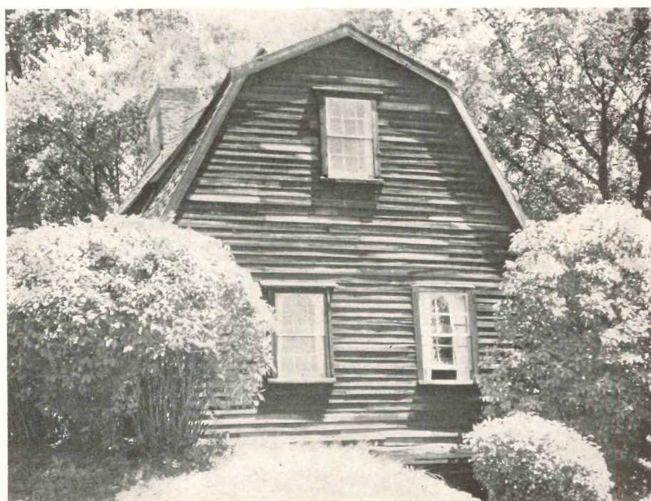
Above: Redwood Inn at Scotia, Calif., with redwood siding and trim on first floor, redwood shingles on the second. It was 20 years old here and had never been painted. Below: the Old Fairbanks House, Dedham, Mass., built in 1636 and never painted. White pine siding was replaced in 1903. Window frame, fascia wood may be the original
