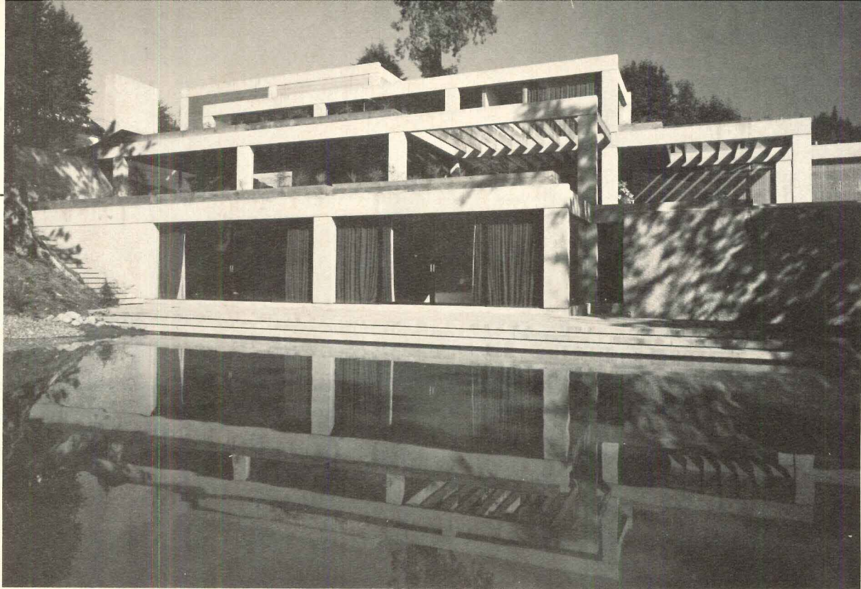
The concrete frames of the Eppich house step down the hillside in three evenly graduated bays. This massing not only reduced the apparent height of the house when viewed from across the pond (photo below) but also makes the end elevations (photo left) conform to the general profile of the site.
