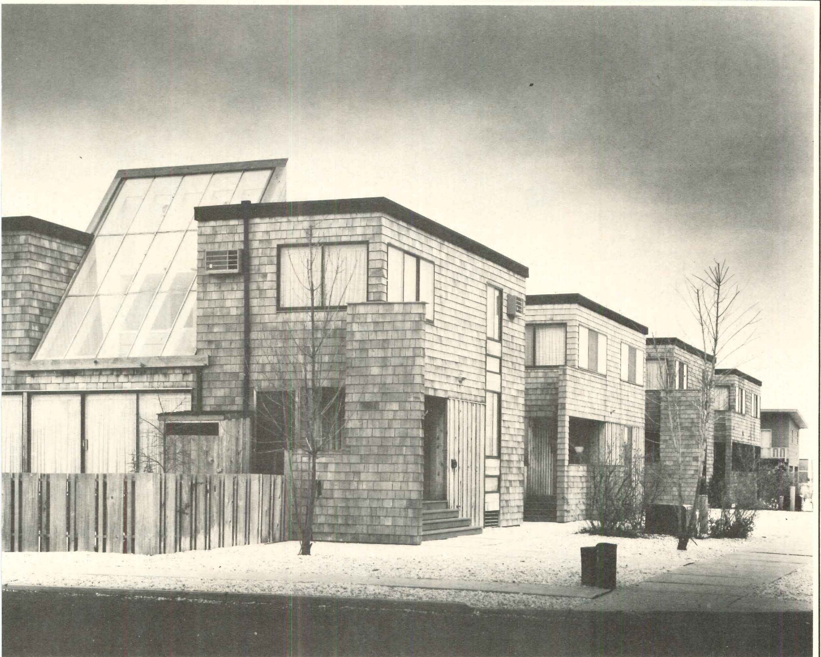
Working with the side yard restriction, Sauer provided each apartment with one blind outside wall (see plan), a design device that protects the privacy of each individual side yard.
