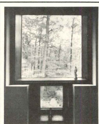
The window treatment (above) reflects the level of design concern. It has a fixed pane for viewing and an operable pane for ventilation.
