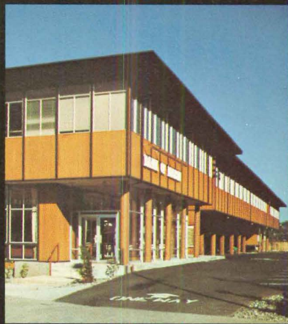
Office Building—Sausalito, California Arch.: Wurster, Bernardi and Emmons, Inc., AIA Structural Engineer: W. B. Clausen
