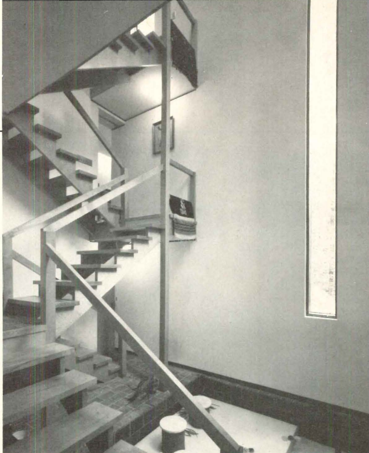
The window treatment (above) reflects the level of design concern. It has a fixed pane for viewing and an operable pane for ventilation.
