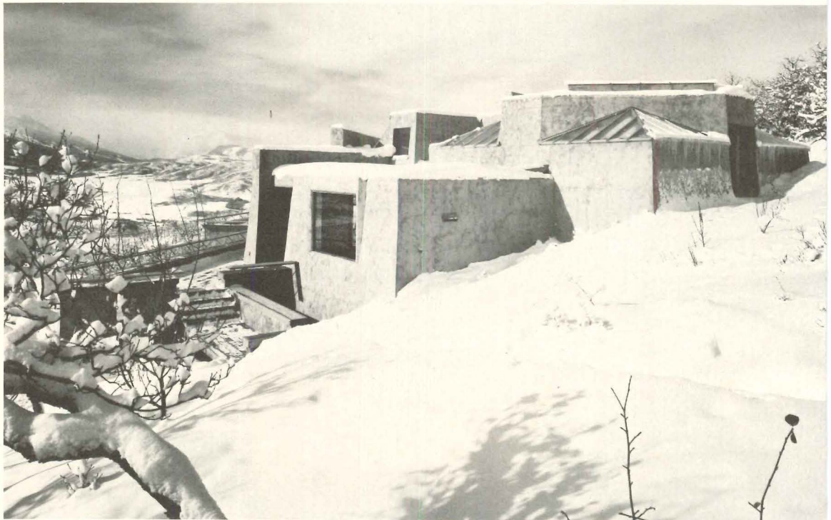
Stucco, over metal channels and lath, is the principal exterior finish. Inside, the owner—who is a painter—required and got large wall display areas of white plaster.
