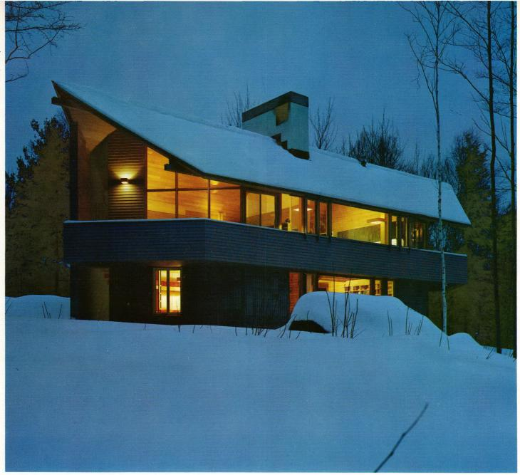
The logical combination of masonry and frame construction gives a crisp clarity to the house (below) and the sheltering roof appears to float above the band of southfacing windows. The massive chimney not only stabilizes the structure but provides a suitablyscaled fireplace. From the built-in couch, skiers can watch the sun set on distant peaks.
