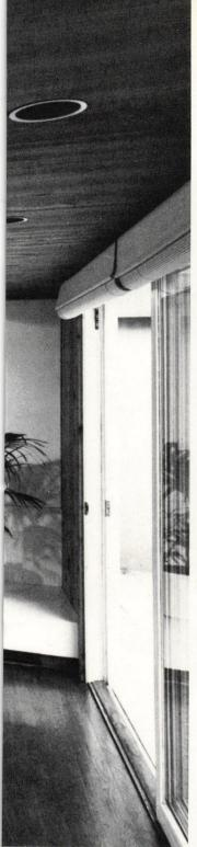
The corner condition, created by the intersection of tilted roof planes over the kitchen (photo right) has been handled with skill. The cabinet partition next to the dining table is kept away from the ceiling while the partition between kitchen and living room reaches full height to provide support for the dropped ceiling over the circulation space as it turns the corner.
