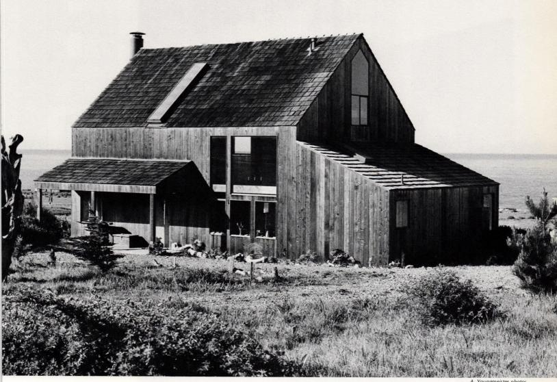
This ingenious vacation house has been built well over a dozen times at the Sea Ranch in California. The basic notion is simplicity itself: a barn-like space with a plan that can be flipped and with an appended lean-to whose function is variable. The working out of the notion, though, assures that simplicity does not lead to dullness.
