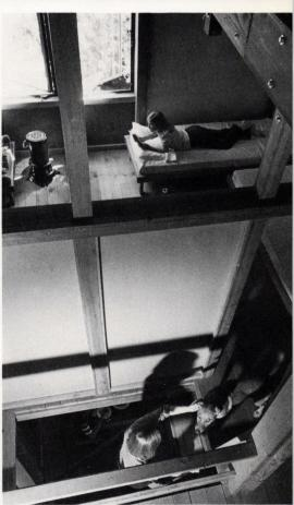
To ease the erection process, Kindorf framed out the floors in doubled 2x6s, bolted in place, and the roof in 2x8s, also paired. Floor planking is white fir, roof is galvanized sheet.
