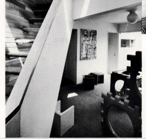
The stairway in the children's wing (left), with open risers and a solid baluster, is a playful switch on usual practice. The white door at the head of the stairs and the one beneath separate the children completely from the rest of the house when that is desired. The parents' bedroom (above) has its own large balcony. It is near the children yet connects, by a bridge, directly to the upper level sitting area in the family-living room wing and to the first floor by the circular stair.
