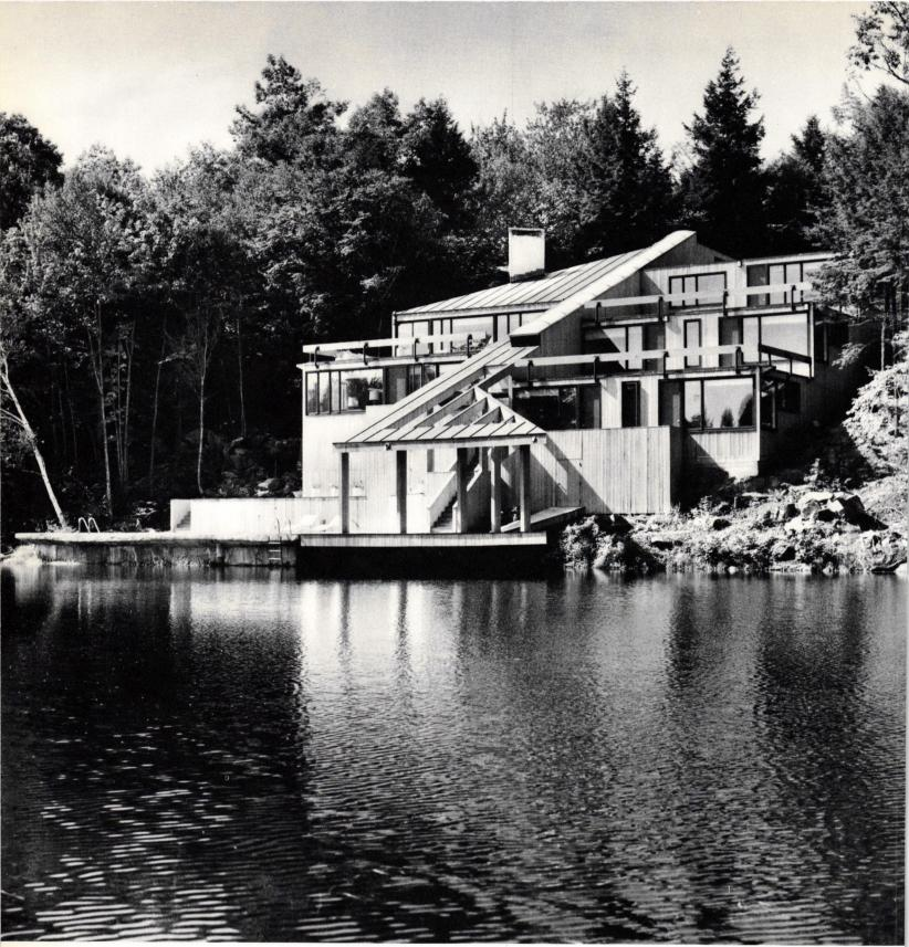
A cool secluded pond is the focus for this house in the Green Mountains of Vermont. Access by car is possible only at a level 35 feet above the water, and so the entrance is at the top and the house is a series of terraced rooms facing the view and arranged around a central stairway that steps down inexorably from the entrance to the pond below, and just before (for the less adventurous) to an open deck and swimming pool.
