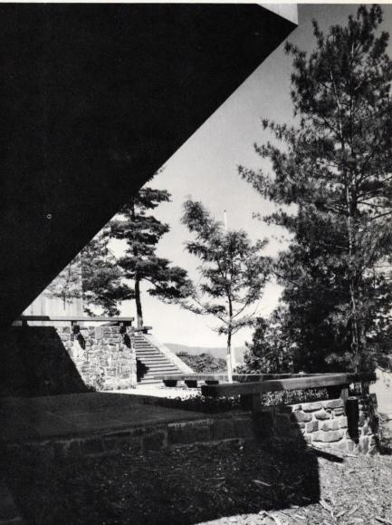
smaller house, which had been destroyed by fire, since building a new foundation would have meant extensive rock blasting and removal from the site. By turning to advantage the oblique angle formed by the existing foundation (see plan) and by cantilevering the main floor over it in both directions (see photo, lower right) the architect was able to gain the added living space required —and increase the drama of the nearly perfect view.
