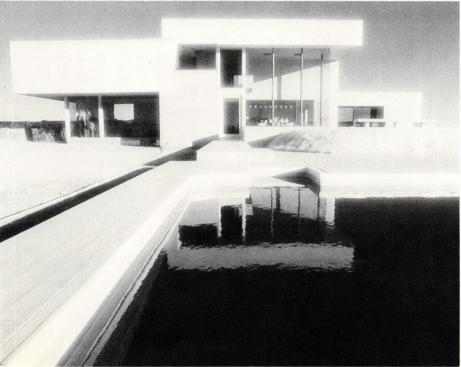
"ong, flat planes of cedar, cantilevered over a stone base" is the phrase Jaffe uses to describe the fundamental concept of this house he designed for the Marvin Schlacters on a flat site in Bridgehampton, Long Island. Here, the ground has been carefully prepared to receive the house. Its mild undulations have been augmented to contrast with the sharp-edged, severely horizontal volumes of the house and to make the ground plane an integral part of the whole composition.
