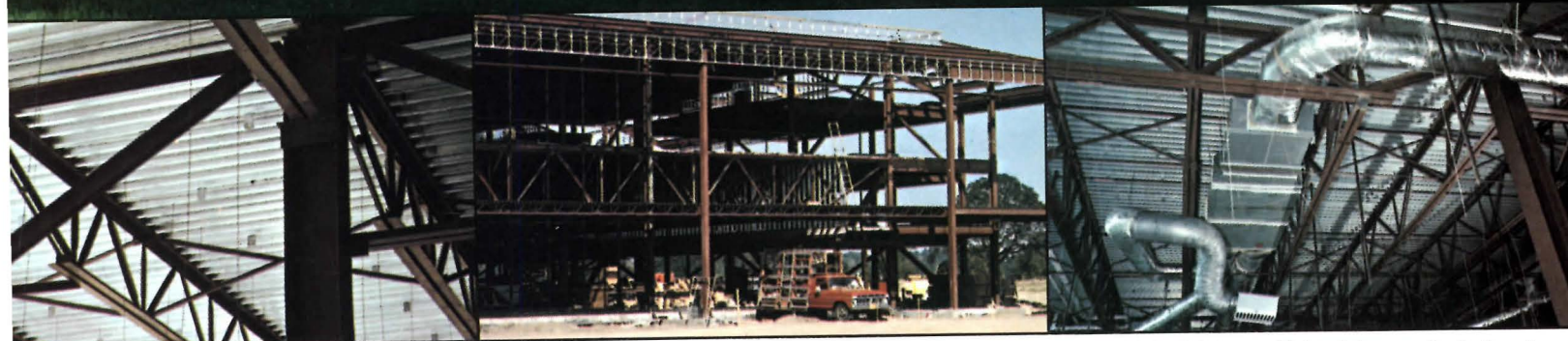
The Hewlett-Packard facility in Cupertino, California, the first of six to use the Vulcraft system.
