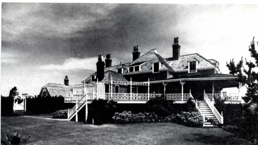
"Sandanwede," a coastal Massachusetts shingle-style mansion, was cited by the jury for "the respect for the existing
