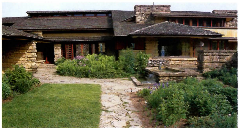
Wright built Taliesin on the side of a hill (top), which turns out to be a slippery slope. The house (above) needs as much as $60 million in renovation work.
