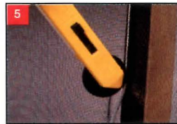
roll screen into base strip
