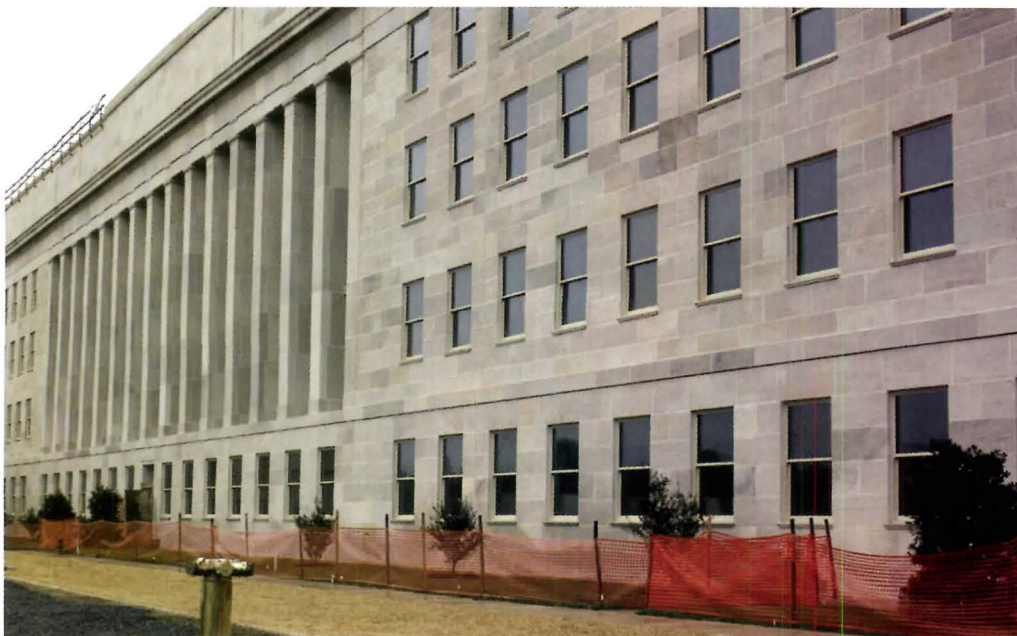
Portions of the limestone exterior of the Pentagon had to be reinstalled following the terrorist attack of September 11, 2001.
