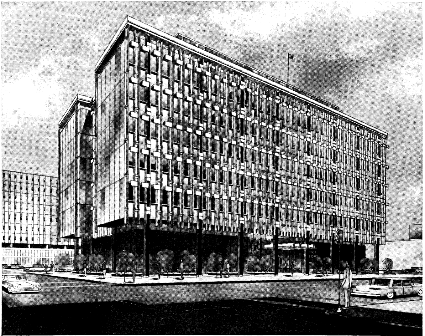
This new Federal Office Building now under construction in Tampa features concrete frame and waffle slab floors complemented by a precast solar skin system with exposed quartz aggregate. Associated Architects are Robert Wielage, AIA, and H. Leslie Walker and Associates with H. Dean Rowe, AIA, as project architect and Dwight R. Abrams as structural engineer.
