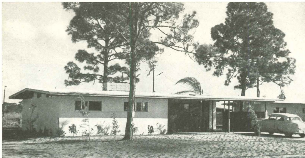
Florida house by St. Petersburg Builder Bruce Wiesemann, Designer Gene Graham, features long, slender design, 1,275 sq. ft. of air-conditioned space for $17,000. Note how wide overhangs shade windows.
