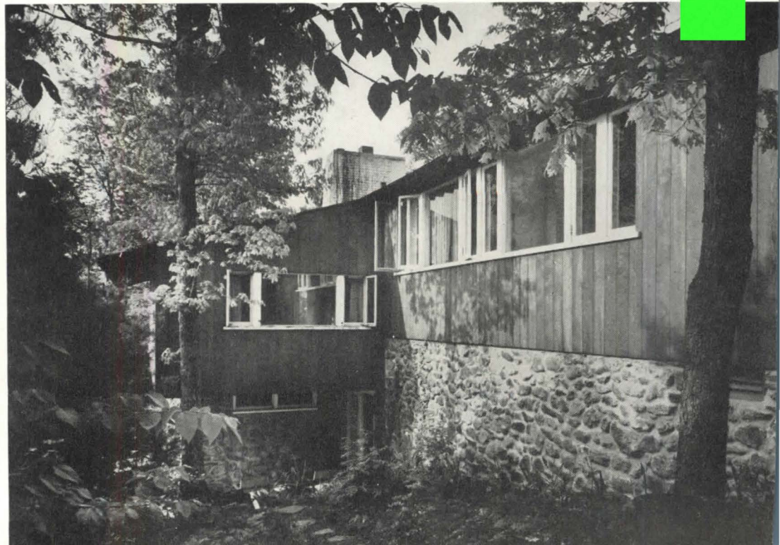
KITCHEN WINDOWS, left; BED-ROOM WING, at right. The house is of frame on fieldstone foundations. Exterior surface is tongue and groove eastern pine.
