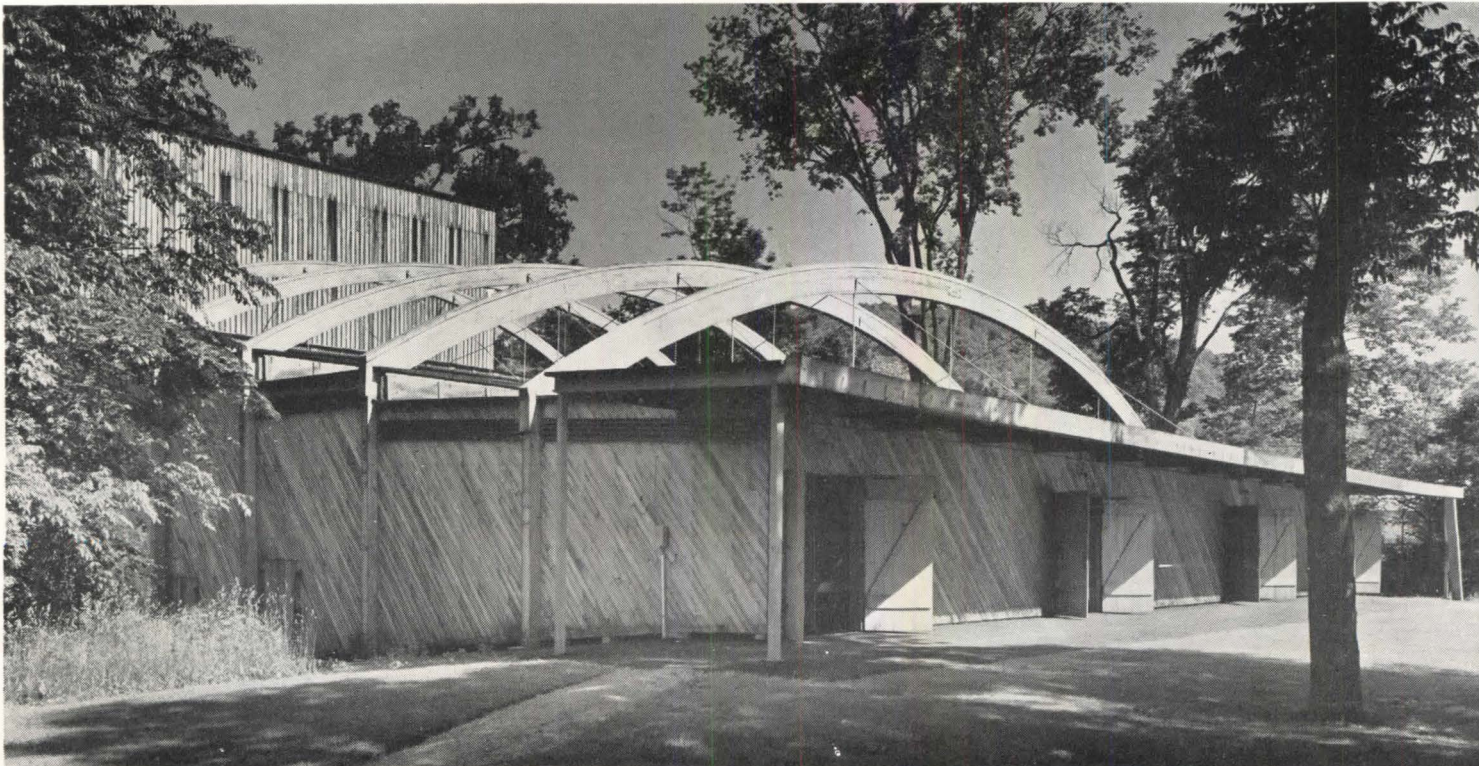
THE PLACING OF THE LAMINATED ARCHES above the roof was necessary "to achieve the right volume for the auditorium."
