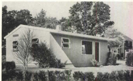
Proved to exceed local code requirements, this prefabricated house was allowed to remain in its Massachusetts setting.
