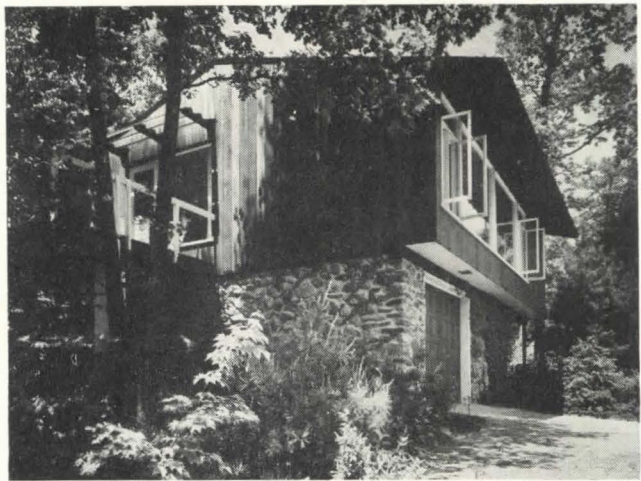
GARAGE AND MAIN ENTRANCE occur at the lower level. By having the garage next to the furnace room, Mr. Oker states, "we get enough heat from steam pipes that pass through the garage to keep it at a temperature much higher than in an unheated garage."
