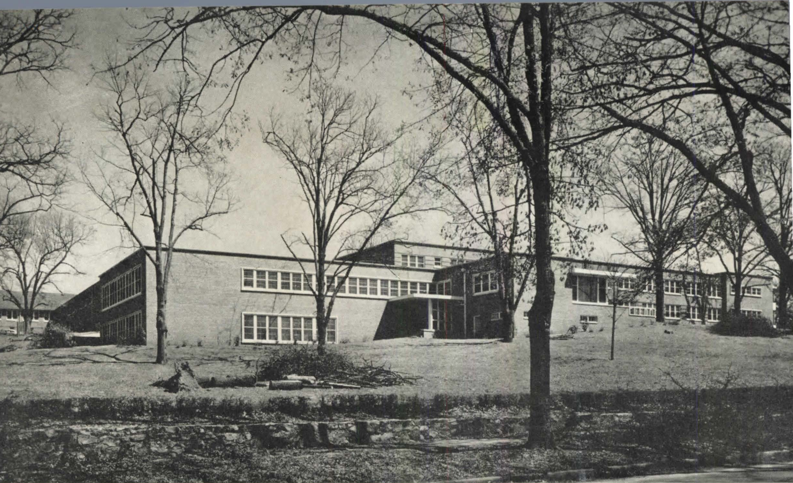
GENERAL VIEW. Hospital in background, at left.
