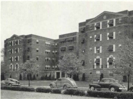
The Lynmore Apartments, Shaker Heights, Ohio. Architect—J. L. Weinberg. Contractor—William Dolin Construction Company.
