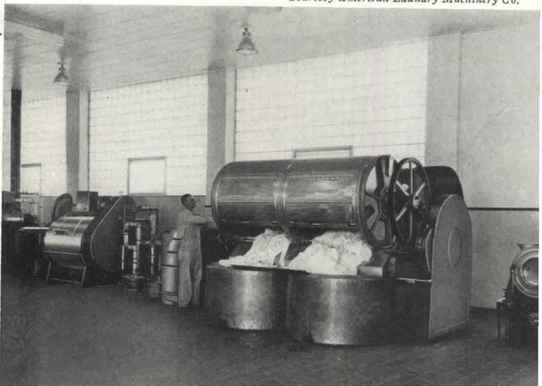
LAUNDRY, O'Connor Hospital, San Jose, Calif., showing automatic unloading washer.
