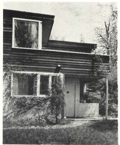
FRONT DOOR. Sitting deck, above.
