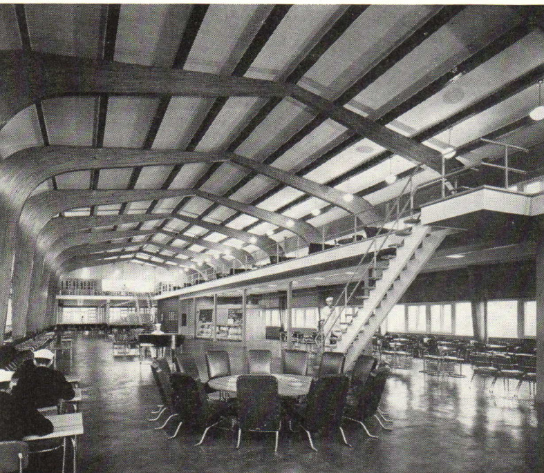
Left: laminated three-hinged arches, acting as both columns and roof supports, are widely used in churches, recreation buildings, and auditoriums. Photo by Hedrich-Blessing; courtesy of Unit Structures, Inc.
