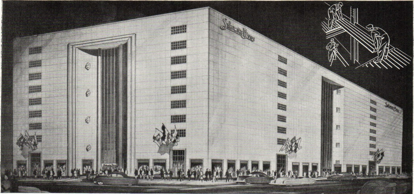
A STORE: Sakowitz Bros. Dept. Store. Tellepsen Construction Co., contractor.
