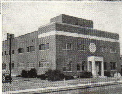
Streptomycin processing and packaging plant built by Merritt-Chapman & Scott for Merck & Company, Rahway, N. J. George P. Butler, Consulting Architect.
