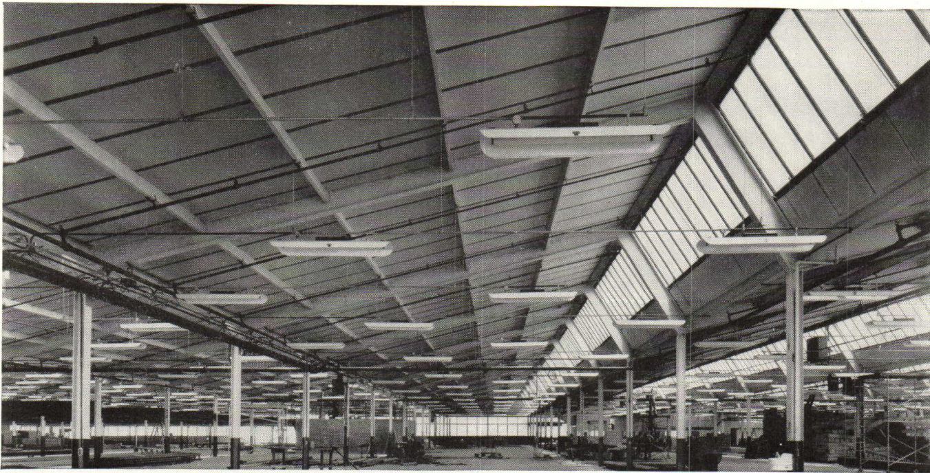
Building for the David Bradley Manufacturing Works of Sears, Roebuck and Company at Kankakee, Illinois ... designed by Sessions Engineering Company. All welded design permitted an unusually low steel weight of 6½ pounds per square foot of area, a saving of two to four pounds per square foot over standard riveted practice.
