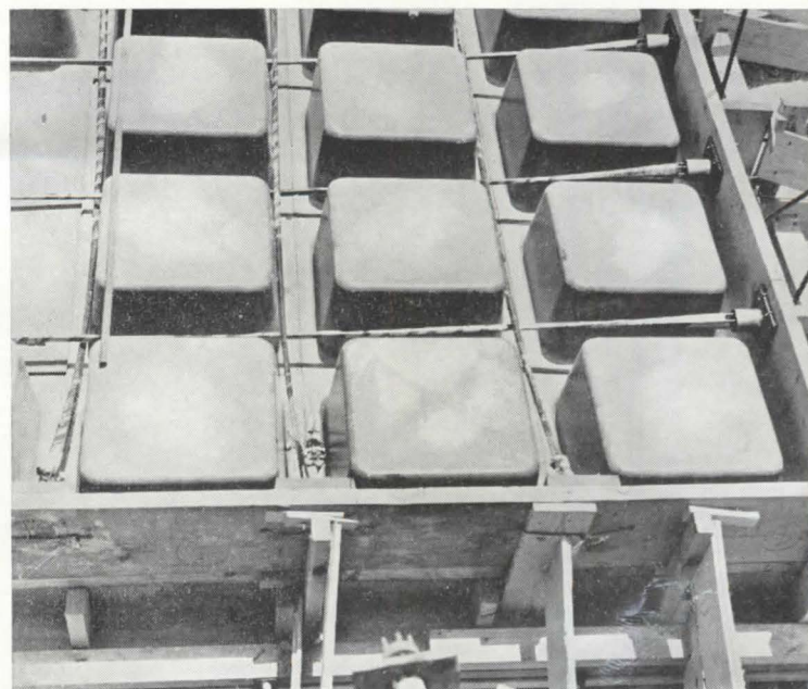
Plastic pans are laid out between edge forms before placement of steel (above). Note absence of pans in shear areas around columns and formwork for opening in slab. Detail photo of prestressing wires in groups (right) shows how end hardware is fastened to forms.
