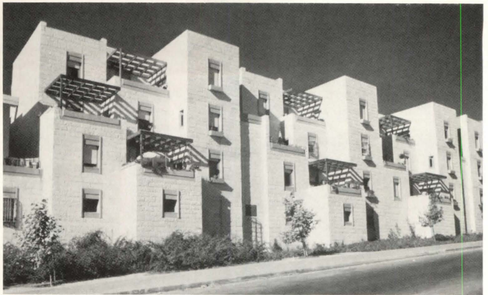
Housing, Ramot Allon: Arie Rahmimoff, architect.
