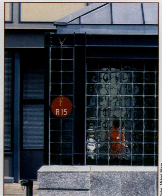
CORNER DETAIL OF ESCALATOR HOUSING
