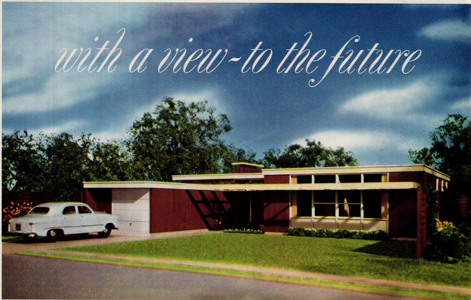
Garage and street side: The facade is varied by the use of setbacks and a two-level roof to avoid monotony. Fence which shields house from street is not shown here. The trellis continues the line of the garage roof and helps tie the two wings of the house together. The outside finish of the Museum-Companion house is of striated Douglas fir plywood.
