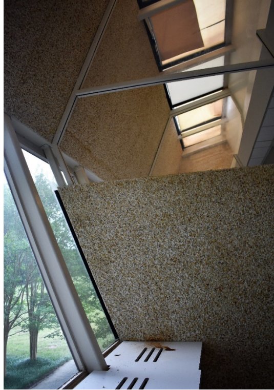
Figure 30: A typical office with access to windows featured not only the main glazing but also a continuous skylight, which posed problems with glare. Author's photograph.
