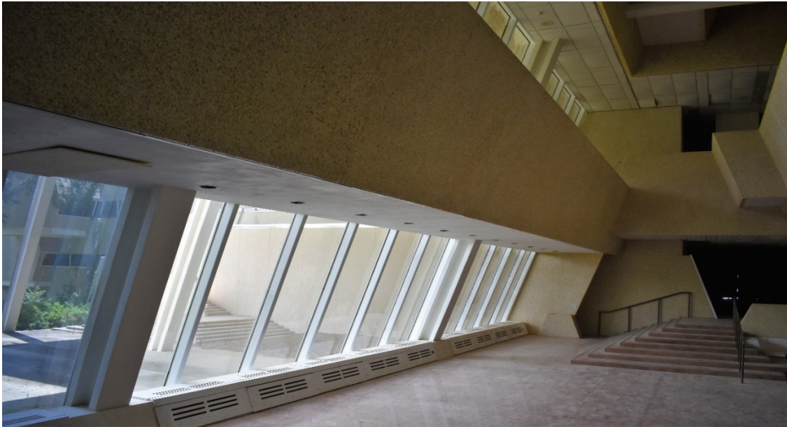
Figure 26: Large continuous glass wall, positioned at a 22.5 degree angle in the lobby of the building. Author's photograph.
