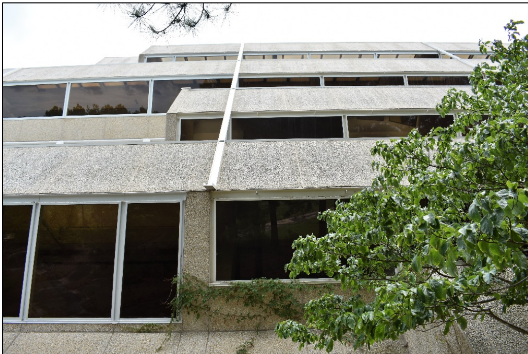
Figure 31: Drainage fits at time awkwardly within the overall design of the Burroughs Wellcome building, for example extending the length of the façade. Author's photograph.
