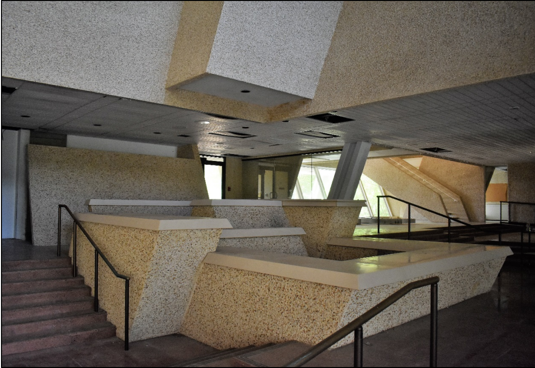
Figure 20: Reception desk at the Burroughs Wellcome building, built using the same aggregate employed in various exterior and interior wall surfaces. Author's photograph.
