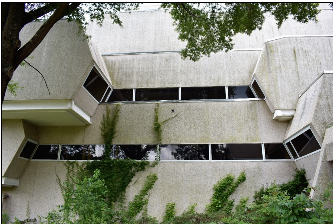
Figure 19: Tinted ribbon windows wrap around a part of the Burroughs Wellcome building. Author's photograph.
