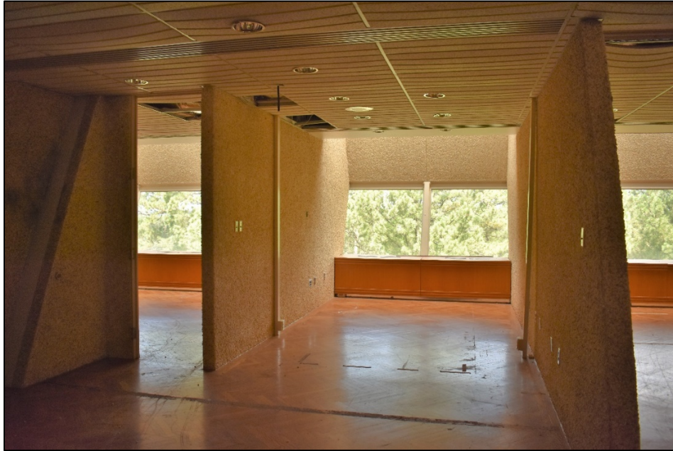
Figure 34: Executive-level offices with open space for secretary space, feature concrete walls floor to ceiling for privacy, whereas typical offices contain a Plexiglas partition at the top to provide more access to natural light. Author's photograph.
